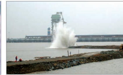
Silt blasting for consolidation in Majishan ore reshipment port
