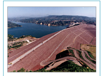
Consultancy on dam deformation control, slope and foundation treatment, and safety monitoring for the Xiaolangdi project
