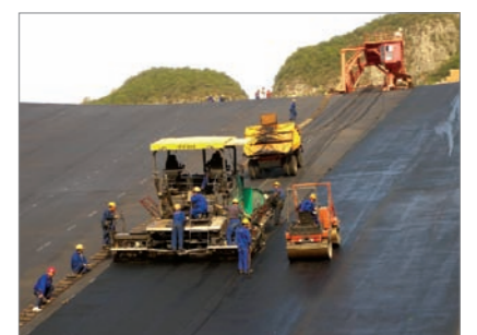
Construction of bituminous concrete facing of the Baoquan pumped storage project
