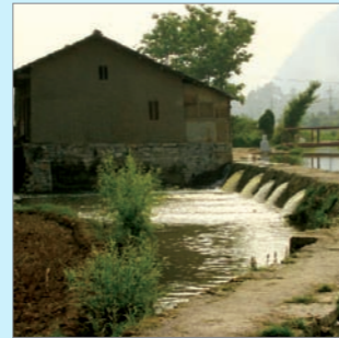
Restoration of the Baotun historical water diversion project
