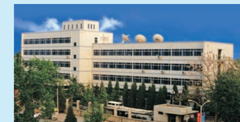
Tianjin Institute of Hydroelectric and Power Research (Tianjin)
