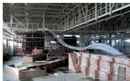
Hydraulic model test of high water head and large discharge spillway tunnel
