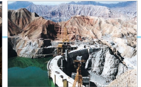
Lijixia Water Project
