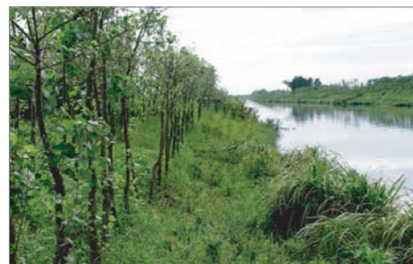
Bank protection with vegetation in rural river restoration
