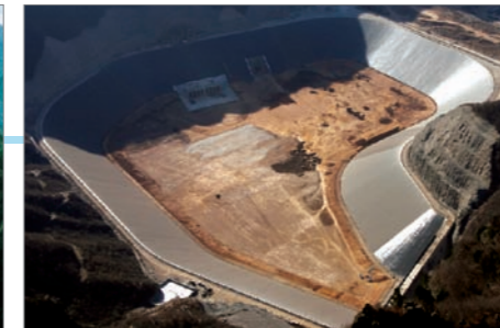
Bituminous concrete faced upper reservoir of the Baoquan Pumped-Storage Power Project
