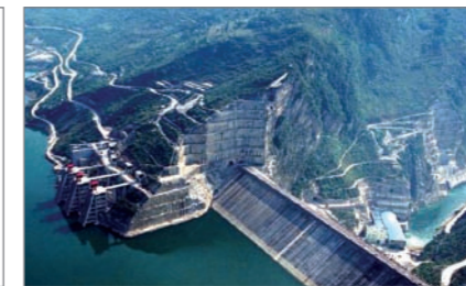
Consultancy on dam deformation control, treatment of abutment slope and water-stop design for the Hongjiadu CFRD
