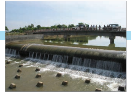
The completed rubber dam in Bangladesh
