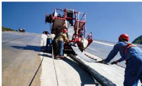
Mechanized installation of GB waterstop materials
