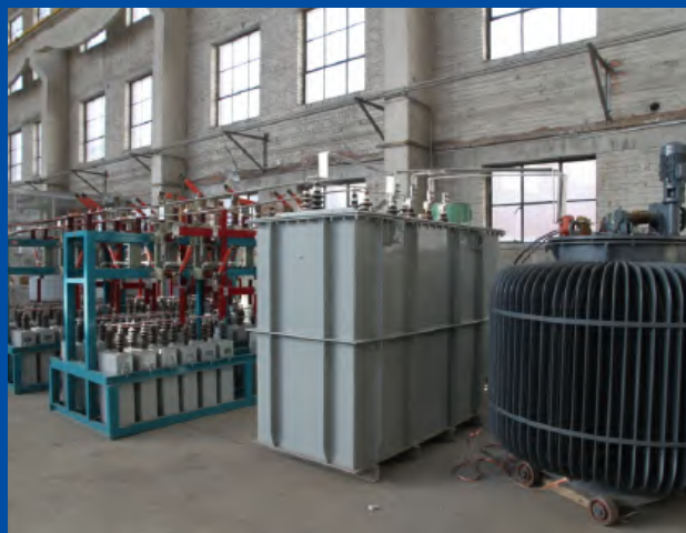
Power equipment testing laboratory
