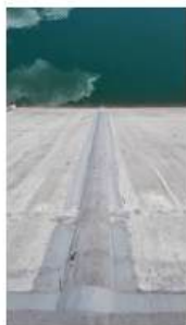
Mechanized installation of GB waterstop materials
