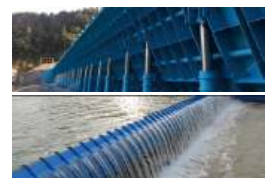
Hydraulic Elevator Dam constructed for purpose of irrigation, landscape, power generation, flood control and flow scheduling
