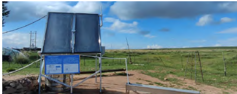
Fig.3 Solar-powered Intelligent Constant-temperature Drinking Water Equipment for Livestock in Baotou City, Inner Mongolia
