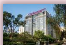
IWHR Headquarter (South)
