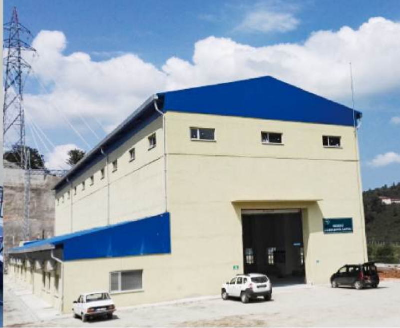
Kozbuku Hydropower Plant in Turkey
